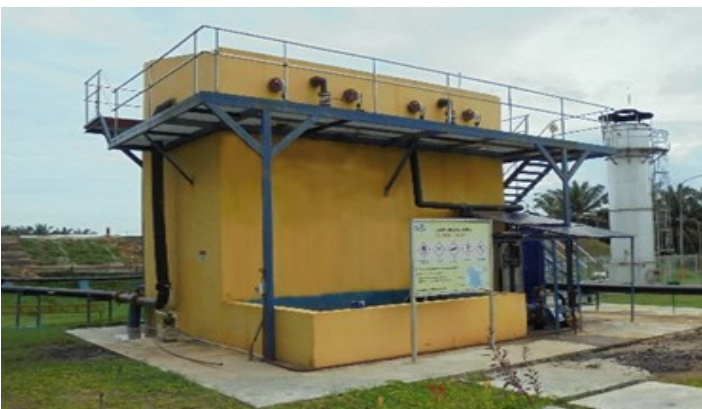
Gambar: Scrubber H 2 S BPO di PT Harapan Sawit Lestari (Sumber-BPO).
