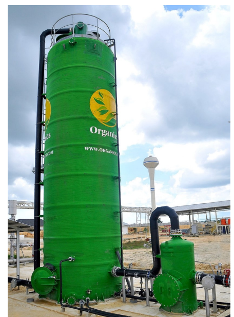
Gambar: Instalasi bio-scrubber Organics Bali (Sumber–PT Organics Bali).
