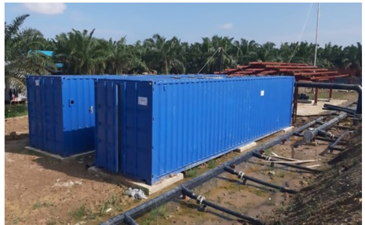
Gambar: Scrubber biologis biogas Elmoz terpasang di PT Pasadena Biofuel Mandiri (Sumber-PT Elmoz Geo Solusi).
